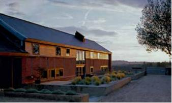
Incorporating large swathes of glazing - for example at gables or in place of the main barn doors - is very popular. These elements will boost natural light, but one downside is they can generate large amounts of rainwater runoff, which increases the risk of damp and decay. The design must therefore incorporate measures to limit the exposure of glazed areas and manage concentrations of runoff.
